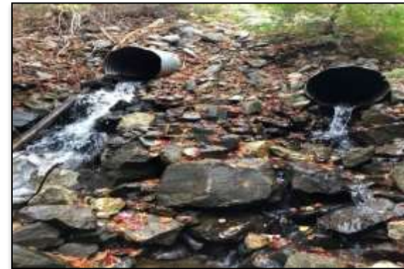
Figure 175. Dual hung culverts do not allow fish passage. Electro-fishing lower stretch and assessing confluence is a priority. Photo: S. Blenis
