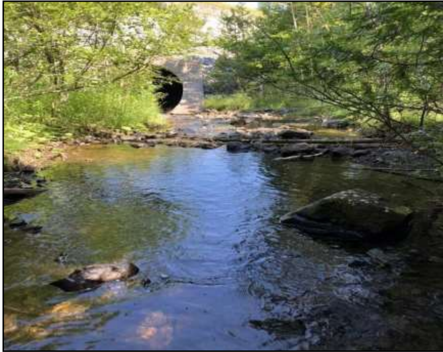
Figure 184. Looking downstream towards the Mackay Highway Photo: J. Kelly
