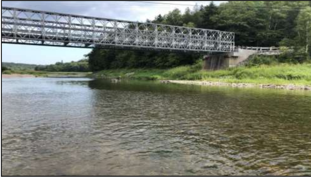
Figure 163. Looking upriver towards the French Village Bridge Photo: S. Blenis
