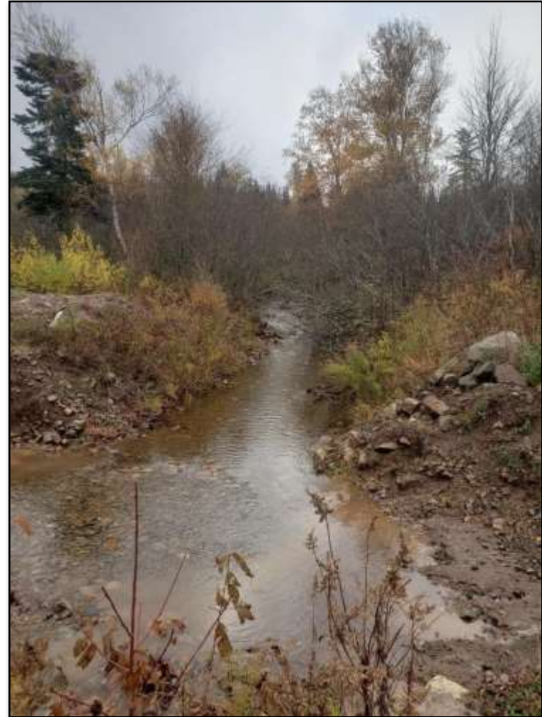
Figure 42. Upstream view of Duffy Brook, showing the degradation caused by trucking through the brook without proper ford, bridge, or culvert. Photo: S. Blenis
