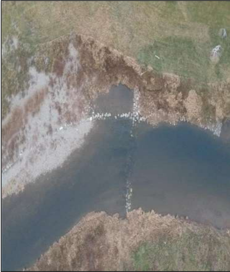
Figure 69. Drone footage from 2020, showing remnants of the 2005 structure, and continued erosion. Photo: M. Adams.
